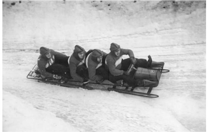
Early bobsleds were similar to wooden sleds used by children. The pilot steers the metal runners in front, and the person in the rear operates the brakes. Credit: German Federal Archive.
