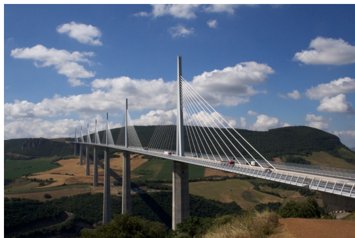
The Millau Viaduct in France is a cable-stayed bridge that crosses a wide valley. Credit: Richard Leeming/flickr.
