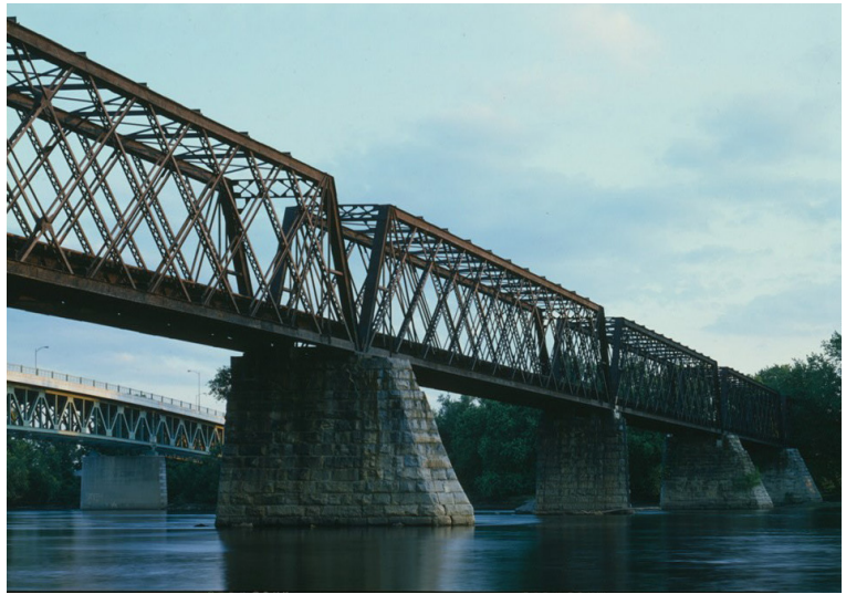
A truss bridge on the Boston & Maine Railroad in Northampton, MA. The bridge was built in 1887 for railcars, but today it is part of a hiking trail.
